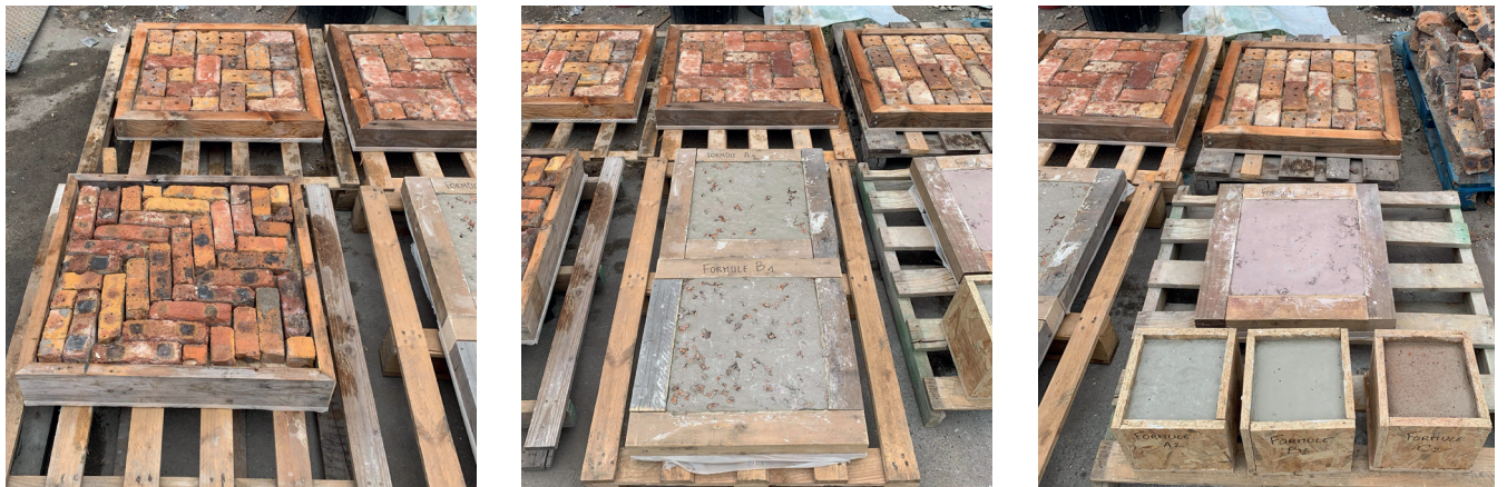
Construction site images: brick assemblies (top), crushing and concrete casting (bottom), Aubervilliers, 2021.
