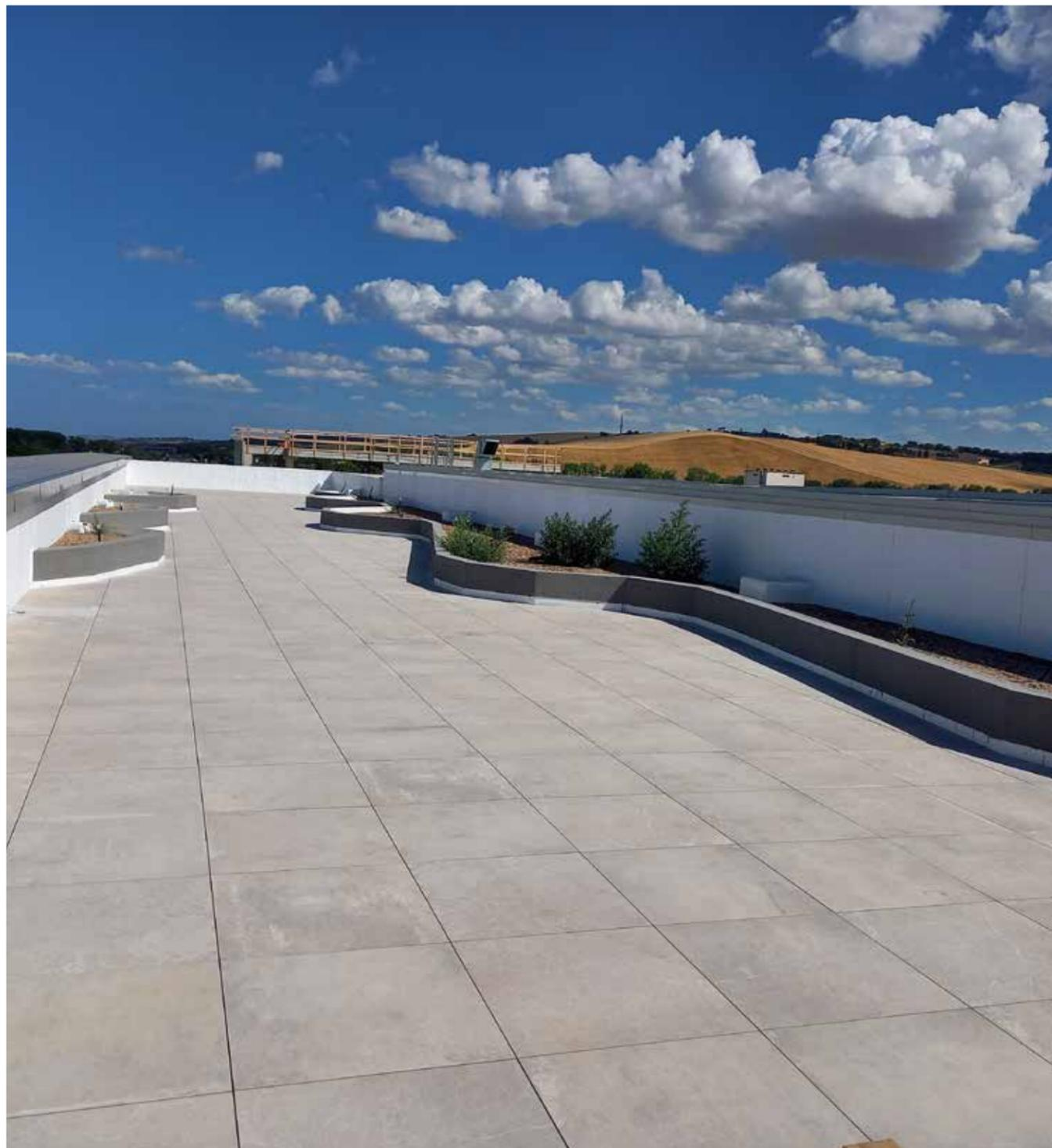
Supply and installation of outdoor raised paving for residential use, comprising GCR body-coloured porcelain stoneware elements, nominal thickness 20 mm, collection and colour to be chosen by Architect and Director of Works, installed dry on an adjustable plastic and metal supporting structure. Module sizes on standard surface 80x80 cm.
